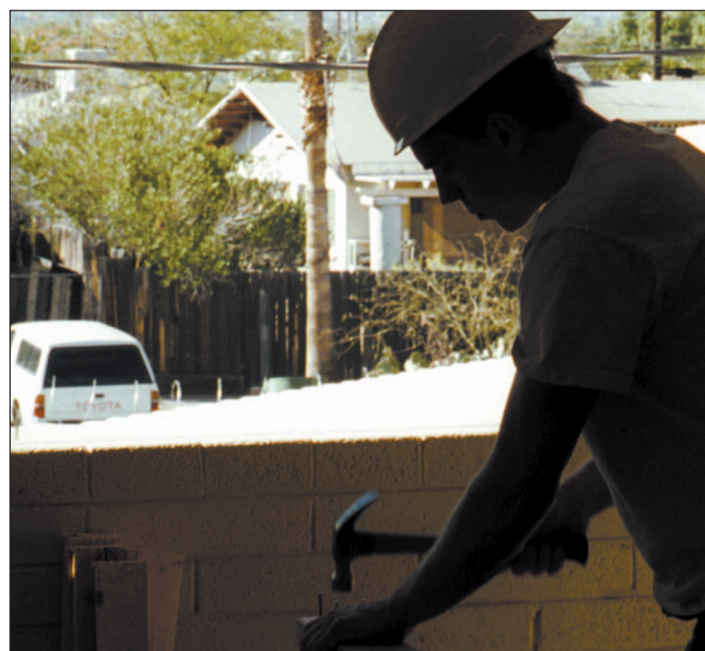
EMILY REID/Arizona Daily Wildcat Carpenter Joshua Morgan works inside the old Sahara Motel Monday afternoon. The Sahara, located on North Stone Avenue, is slated to become private dorms for UA and Pima students.
