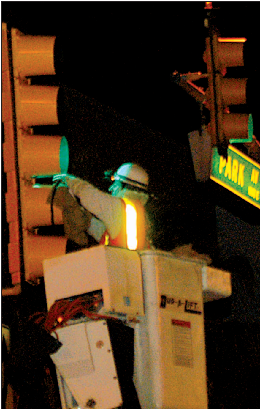
BRETT FERA/Arizona Daily Wildcat City of Tucson employee John Wills, 38, installs the left-turn arrow lamp at the intersection of North Park Avenue and East Speedway Boulevard early this morning. Nighttime work will continue at the intersection until the project is completed.
